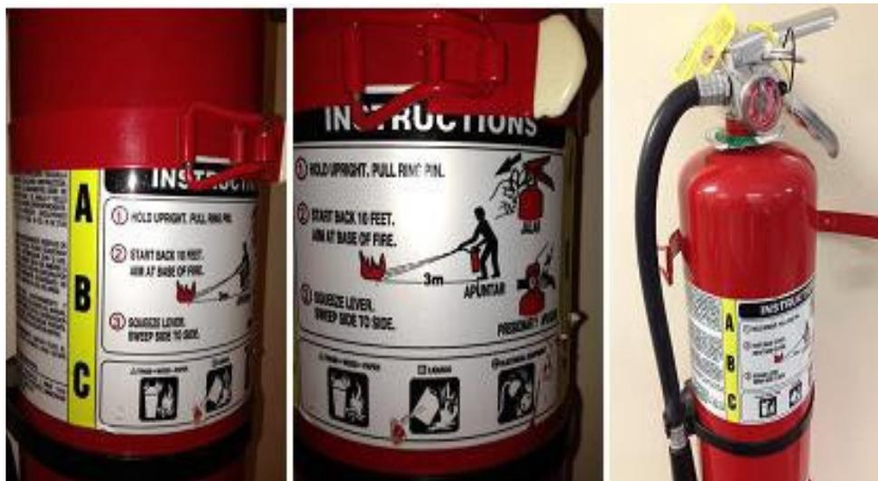
Class A portable fire extinguishers are available but are not as prevalent as Class ABC extinguishers. Class A PFEs are also known as Air Pressurized Water (APW) fire extinguishers. Water is an extinguishing agent for regular combustibles.
