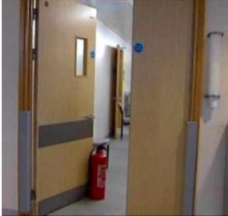
Fire doors illegally propped open with a portable fire extinguisher
