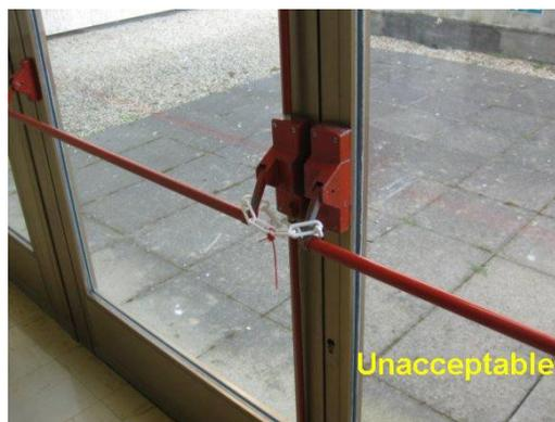
Picture shows a chained exit door, which is unacceptable.
