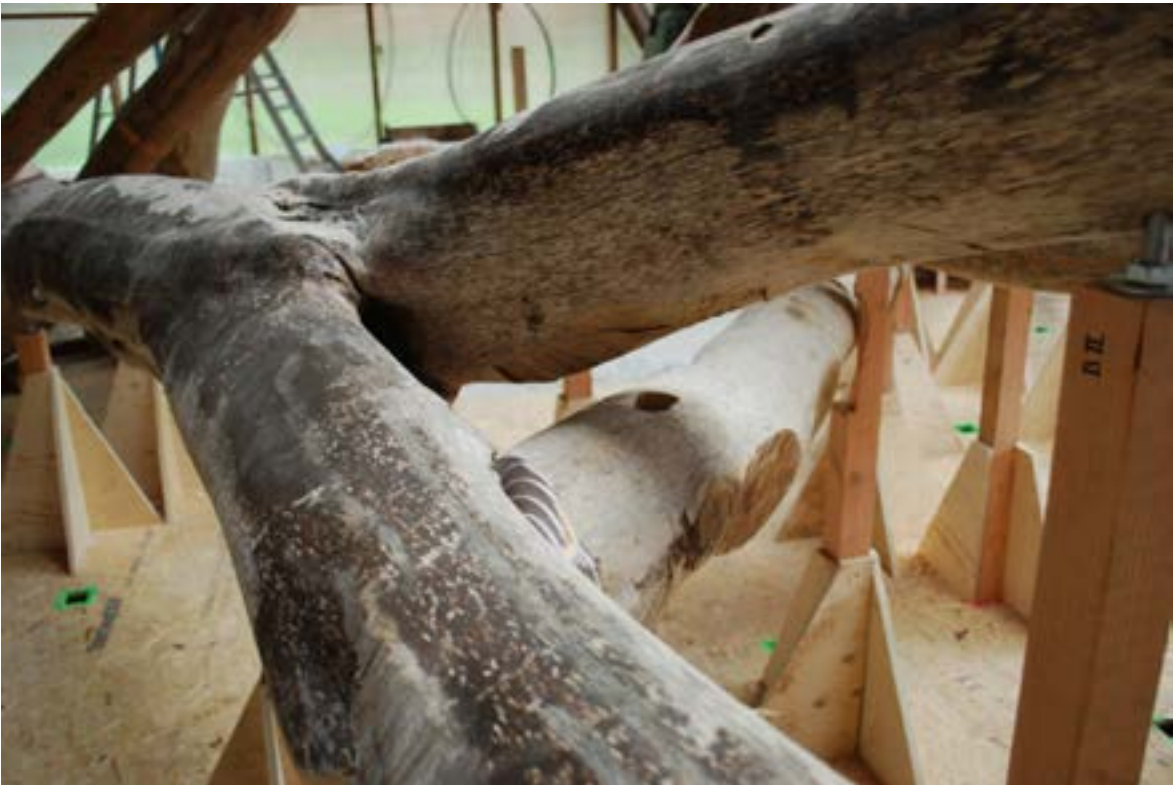
Fig. 23. In a number of cases, forks pass by each other with little room to spare. Once assembled, most traces of robotic fabrication are concealed.
