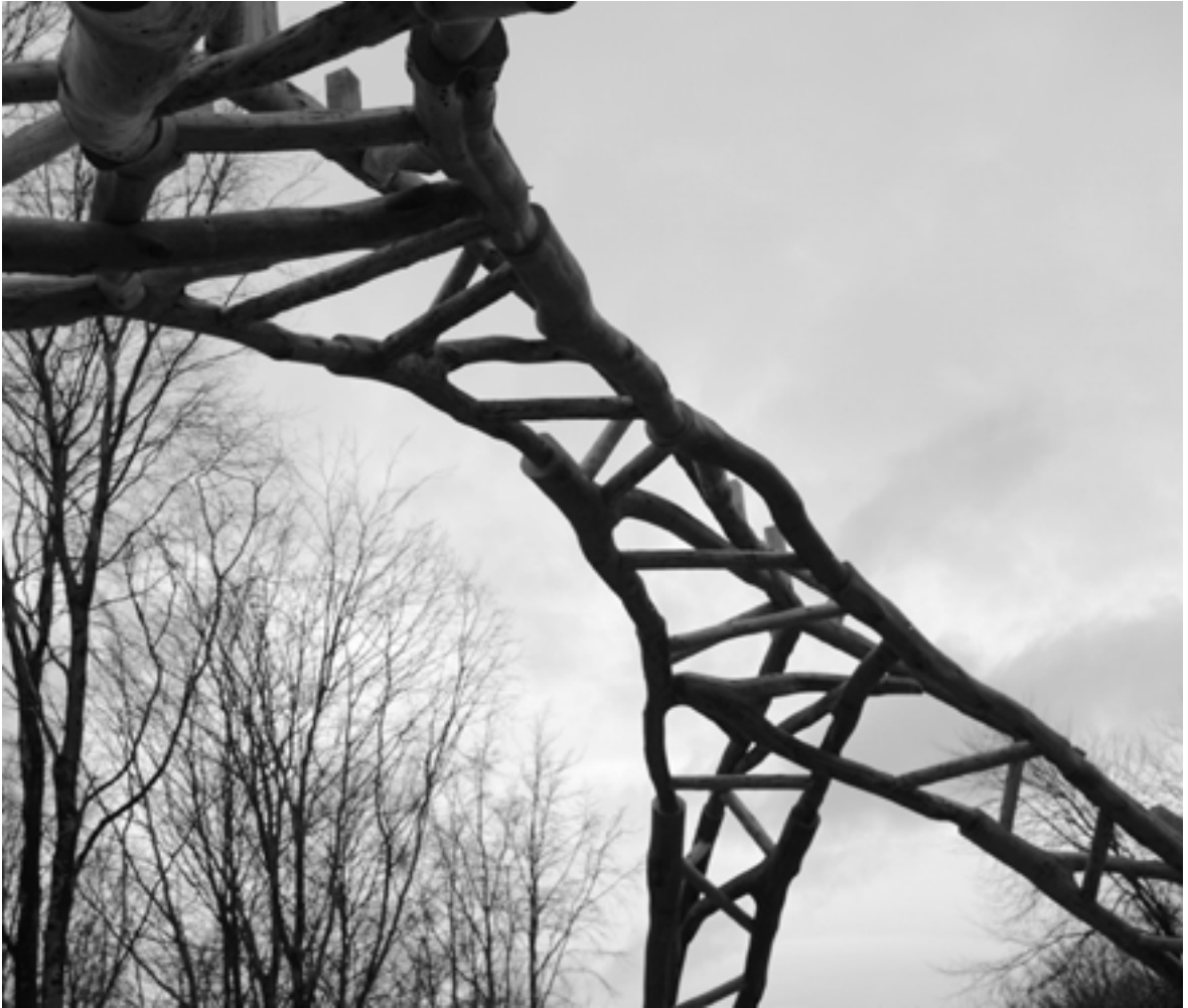
Fig. 25. The Tree Fork Truss
