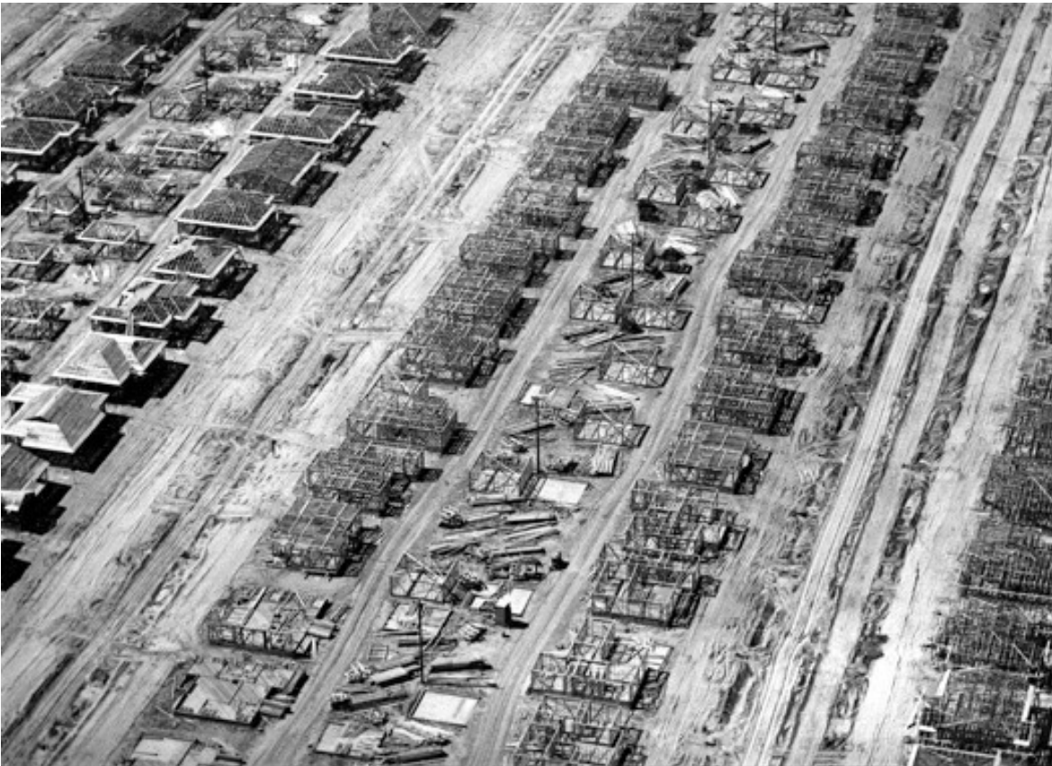
Fig. 3. Counter to the sensitive use of wood by early craftsmen, this aerial photo shot in 1950 by William Garnett shows the change to building systems based on standardized materials under mechanization.
